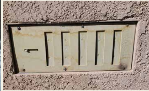
Close crawl space vents in the winter.
